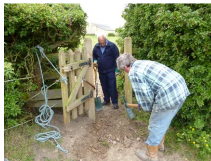
Risley FP16 – levelling off for stoning
