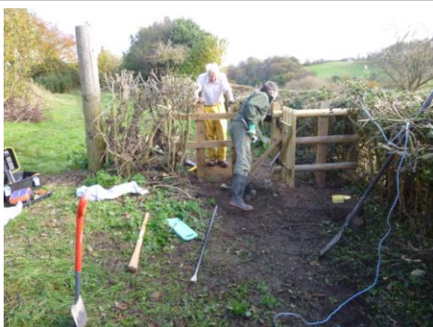
Fencing in progress
