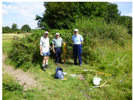
Way marker post installation team – Dale Abbey FP26
