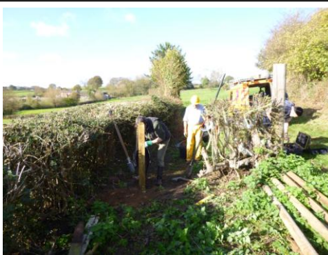
Site cleared, hinge post in place
