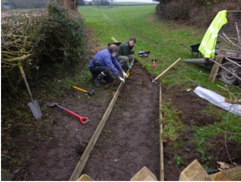
Clearing ground and setting out
