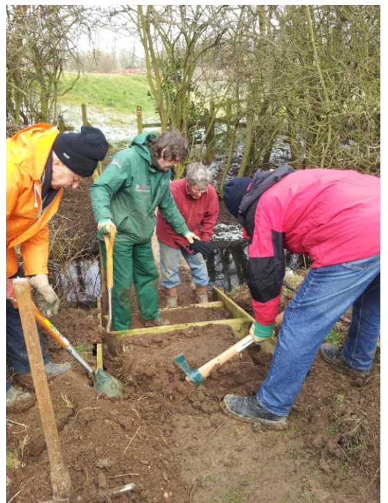
Step work in progress
