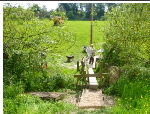
Stone raft completed
