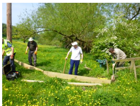
Laying out causeway
