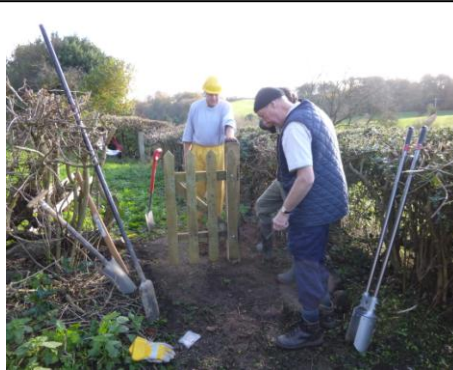
Gate hung ready for slam post
