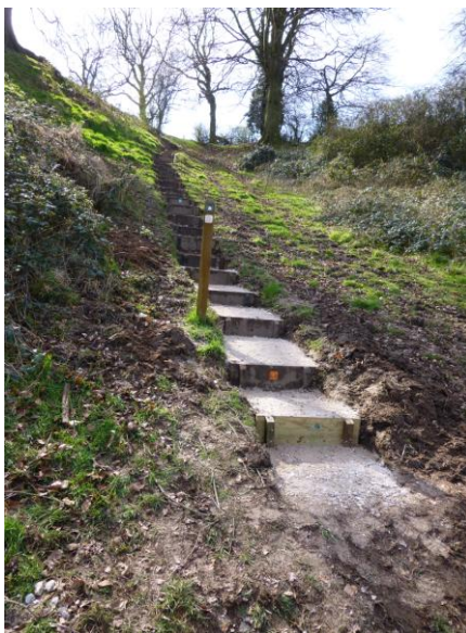
Stoning of steps in progress
