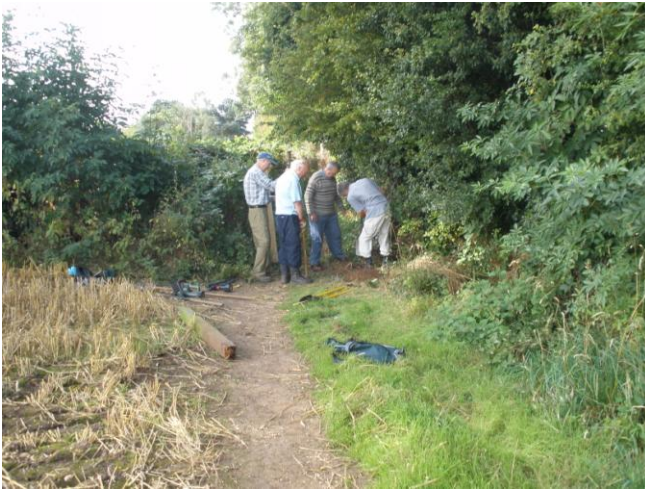
Ockbrook FP13; Preparing problem ground for new waymark post
