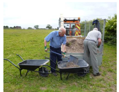
There was a lot of barrowing of stone to sites to be done
