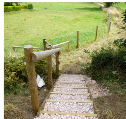
Phase 1 of step replacement completed
