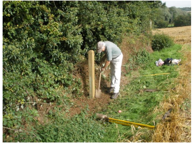
Ockbrook FP13/14; tamping in new waymark post
